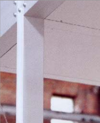
The ceiling elements are slotted into the suspension profiles.
