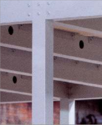
Ceiling supports with openings for cable and service ducts.
