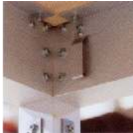
The flooring elements are bolted to the support brackets.
