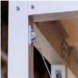
Cross bracing ensures stability and safety.
